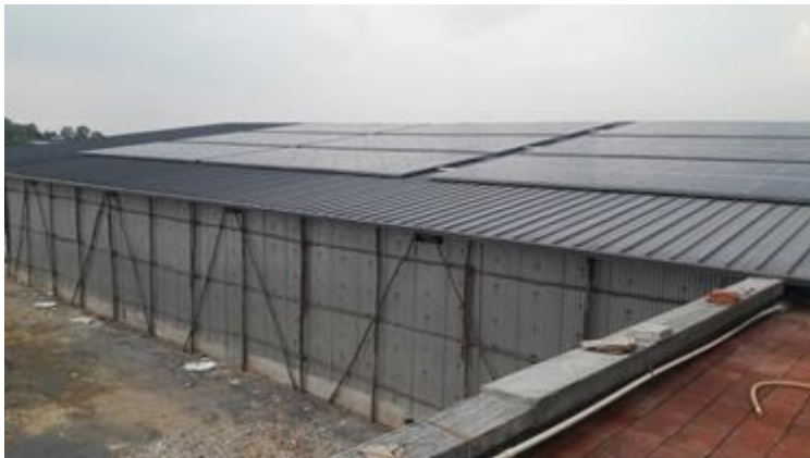
SEZ Studio-1 Solar Panel
